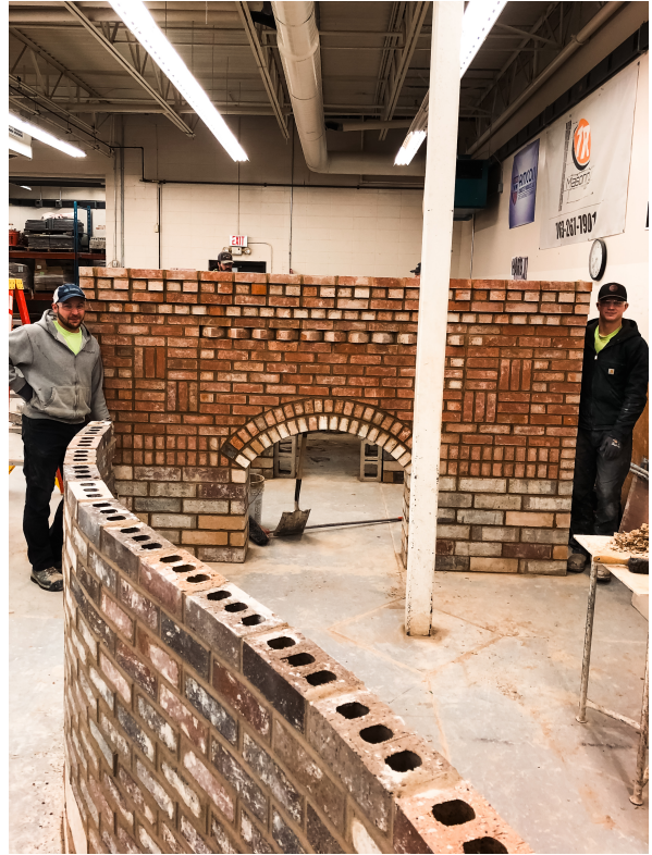
3rd Year Apprentices Jeremiah Jones and Riley Strate pictured with their arch project and serpentine wall.
