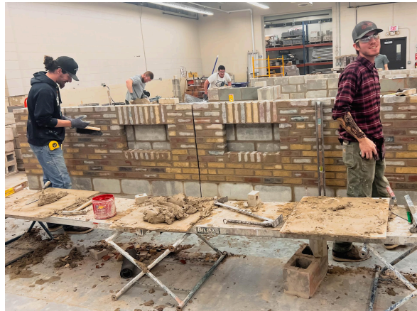
1st Year Correspondence Brick Apprentices Brock Lizotte and Darrin Aleckson working together to build a brick and block window wall project.
