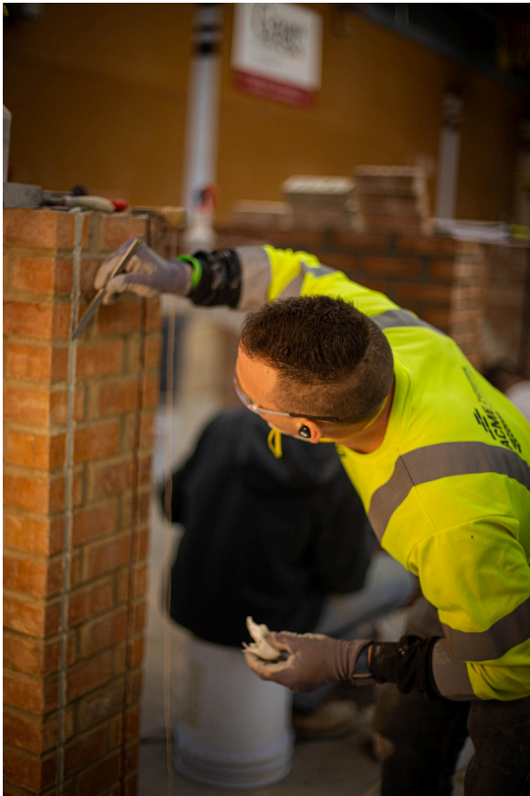
1st Year PCC Apprentice Chad Lee practices caulking.
